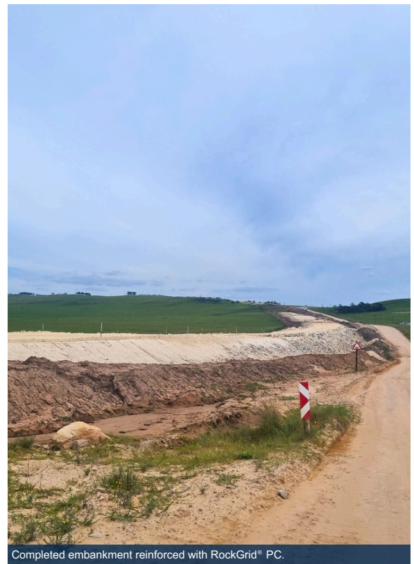
Completed embankment reinforced with RockGrid® PC.
