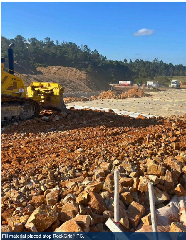
Fill material placed atop RockGrid® PC.
