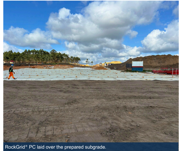
RockGrid® PC laid over the prepared subgrade.
