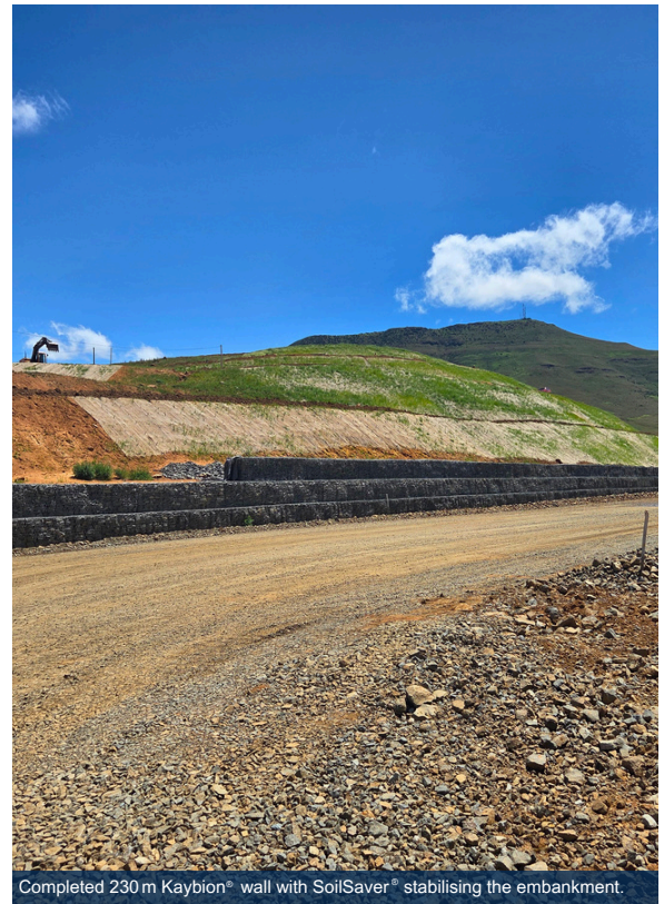
Completed 230m Kaybion® wall with SoilSaver® stabilising the embankment.
