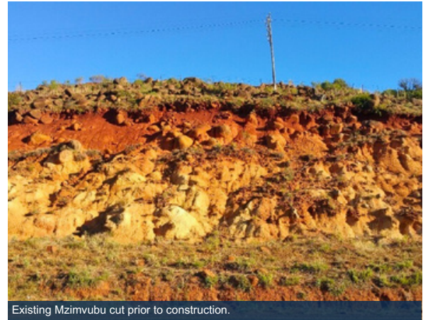
Existing Mzimvubu cut prior to construction.
