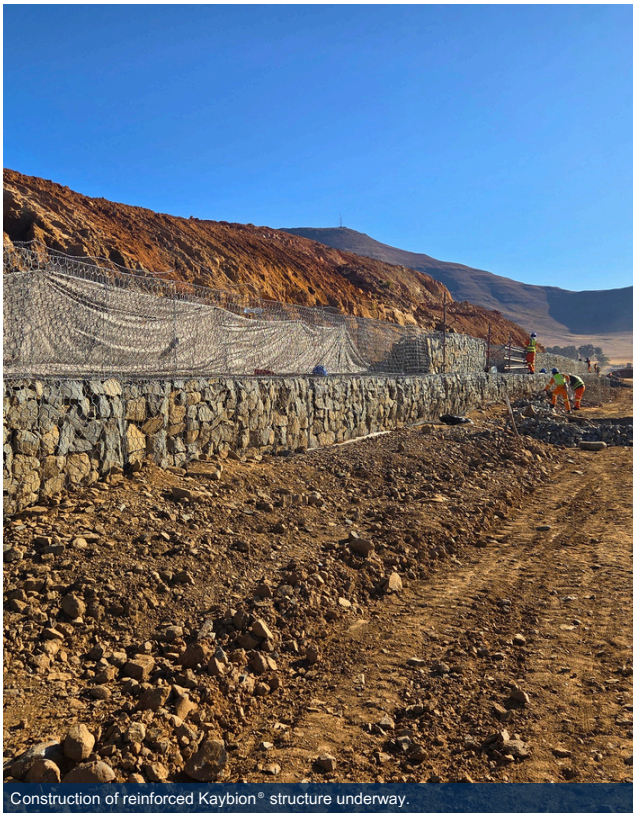
Construction of reinforced Kaybion® structure underway.
