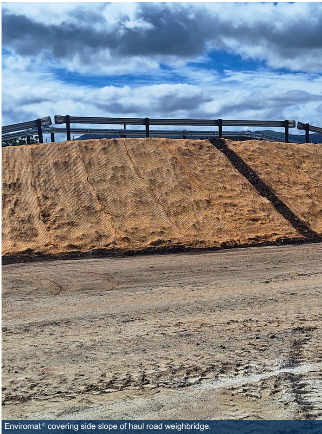
Enviromat® covering side slope of haul road weighbridge.
