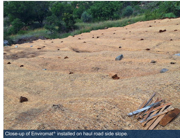
Close-up of Enviromat® installed on haul road side slope.
