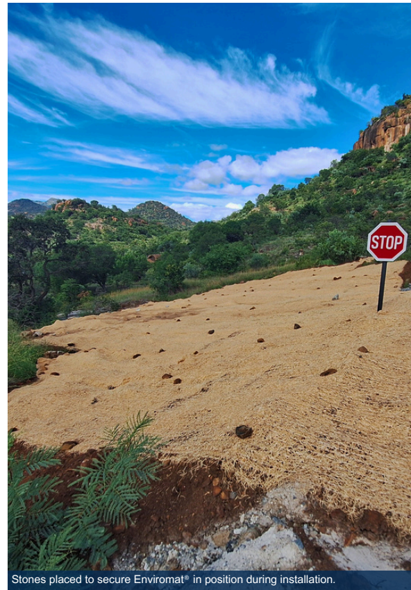
Stones placed to secure Enviromat® in position during installation.
