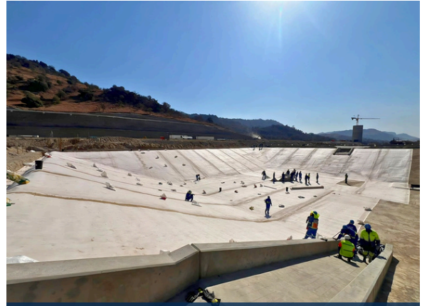
EnviroFix® positioned on the dam base to form the secondary containment layer.
