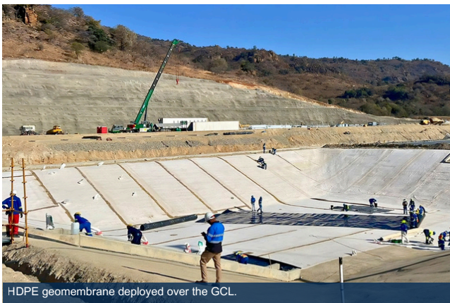
HDPE geomembrane deployed over the GCL.
