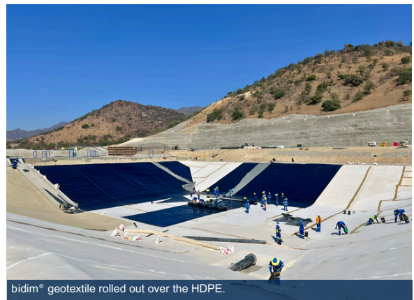
bidim® geotextile rolled out over the HDPE.
