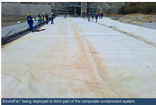
EnviroFix® GCL pulled into position prior to installation.
