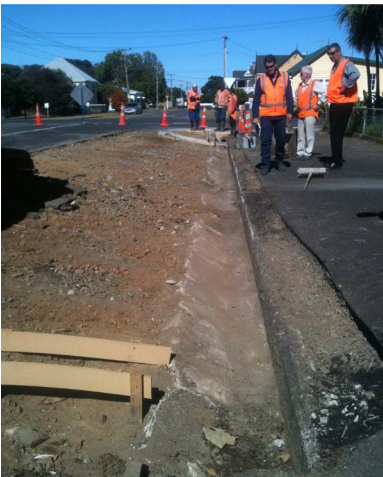
Original concrete curb
