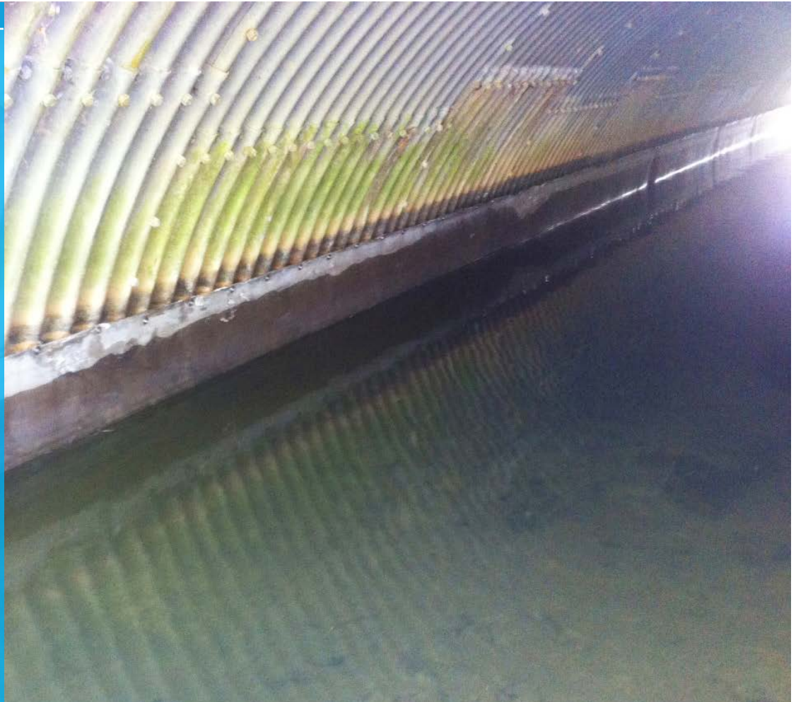
The completed project
