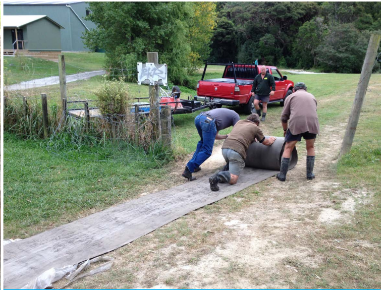
Unrolling the CC8™ to cut it to length
