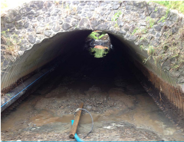
The culvert before work began
