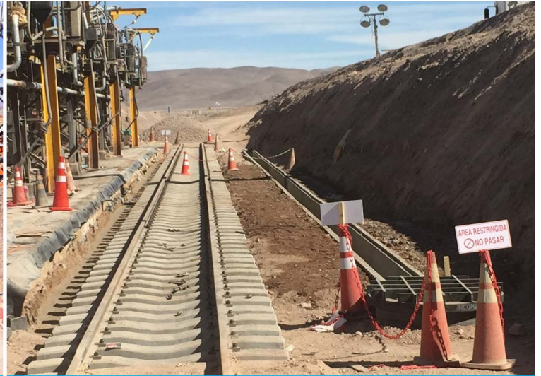
First pre-cast concrete ditch installed
