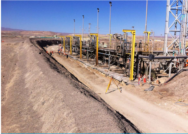
Site just after works began
