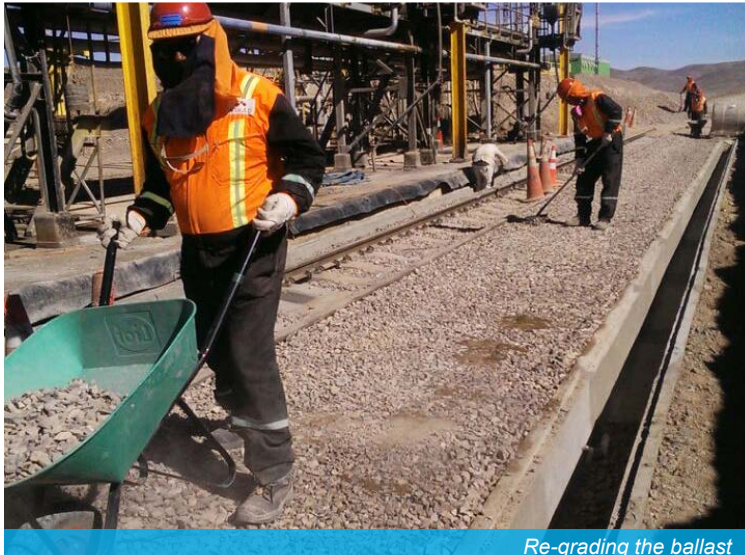
Re-grading the ballast
