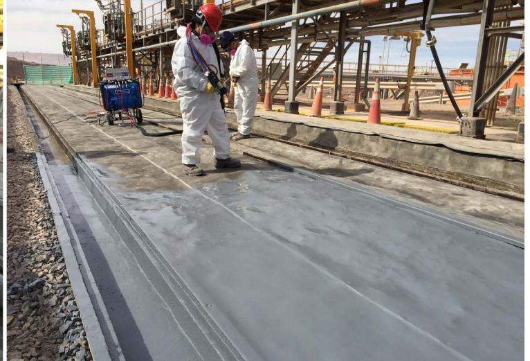
Applying the polyuria layer
