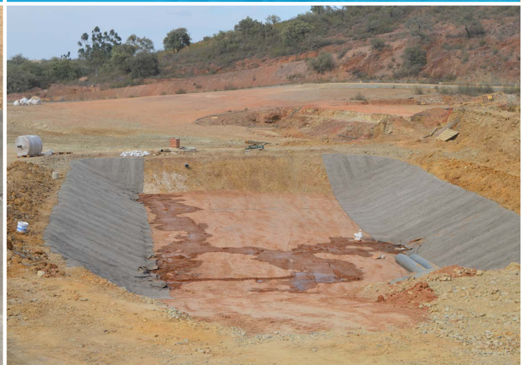
Completed sections on the longest sides
