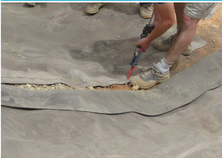
Applying Everbuild Clearfix sealant
