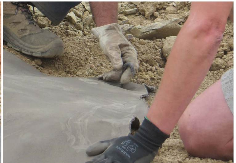
Pegging the CC into the anchor trench
