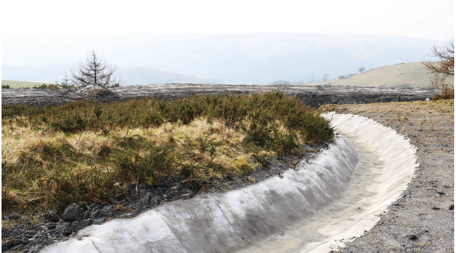
Phase 2 completed transverse corner section of ditch
