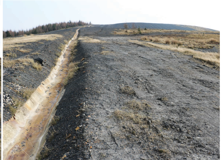
Channels show no signs of degradation and no requirement for maintenance
