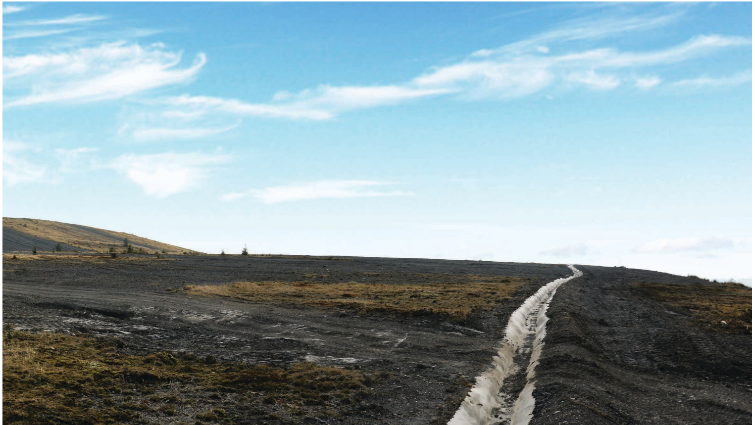
Phase 2 completed longitudinal section of ditch
