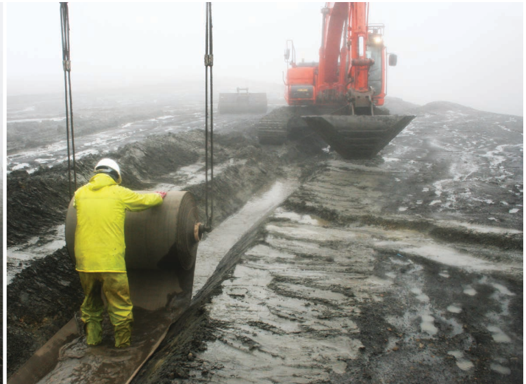
Phase 1 CC13™ Bulk Roll deployment in challenging weather conditions
