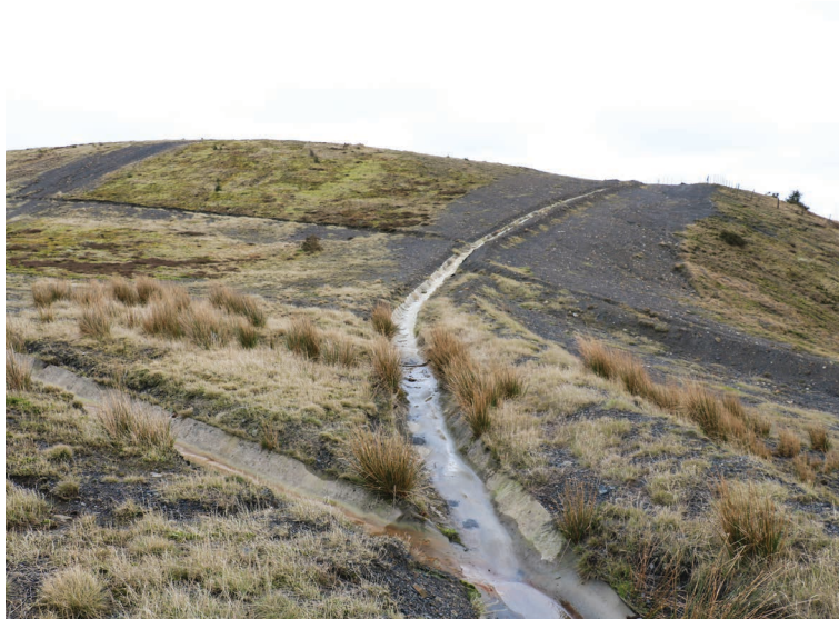
Phase 1 intersection 5 years after installation
