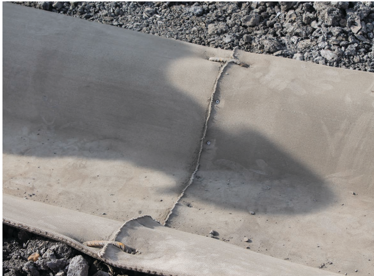
Longitudinal overlap detail
