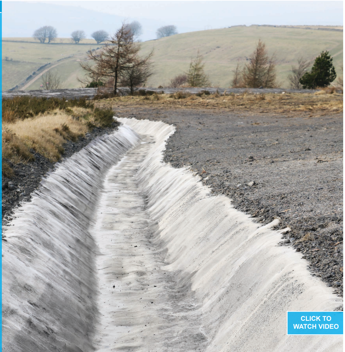
Completed CC lined drainage channel
