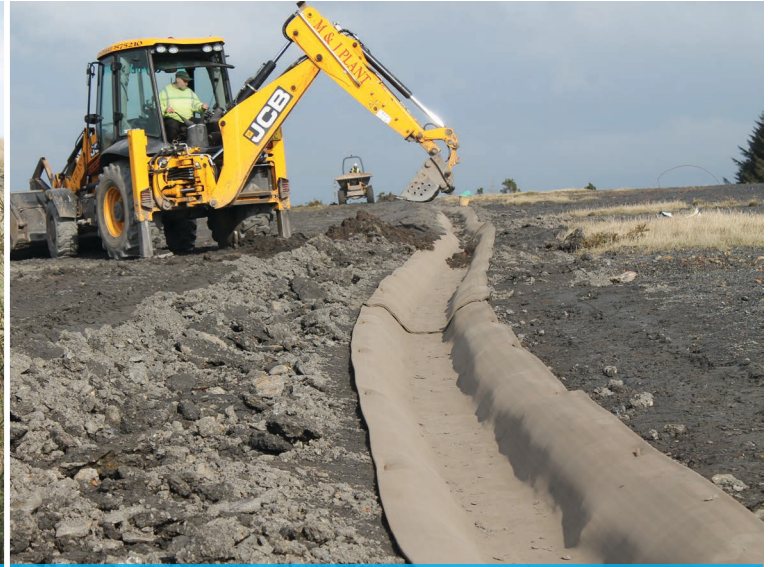
Phase 1 longitudinal lining
