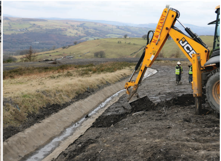
Backfilling
