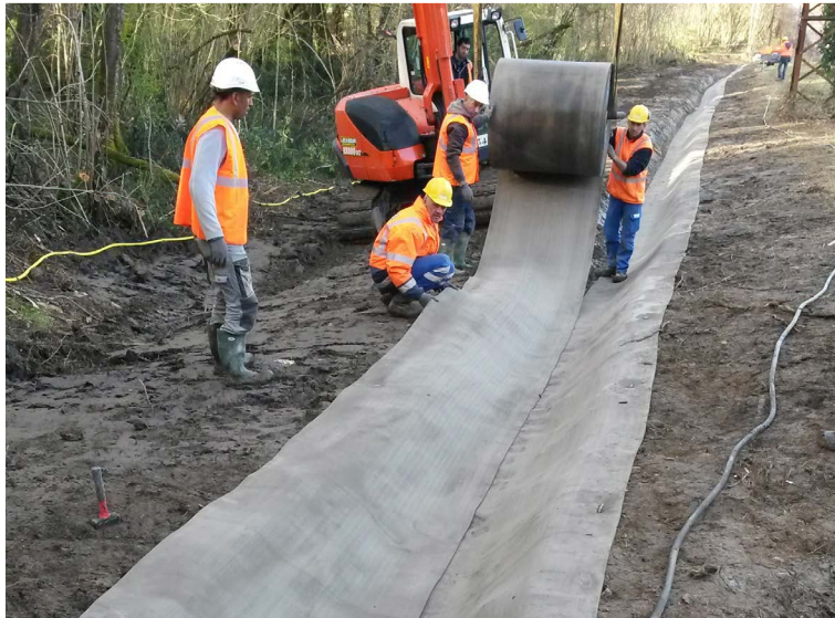
Unrolling the second layer of CC
