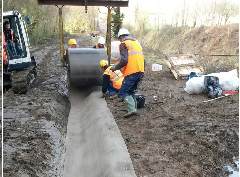
Unrolling the first layer of CC
