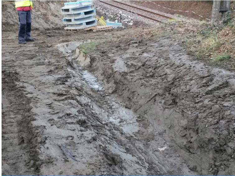
The graded ditch
