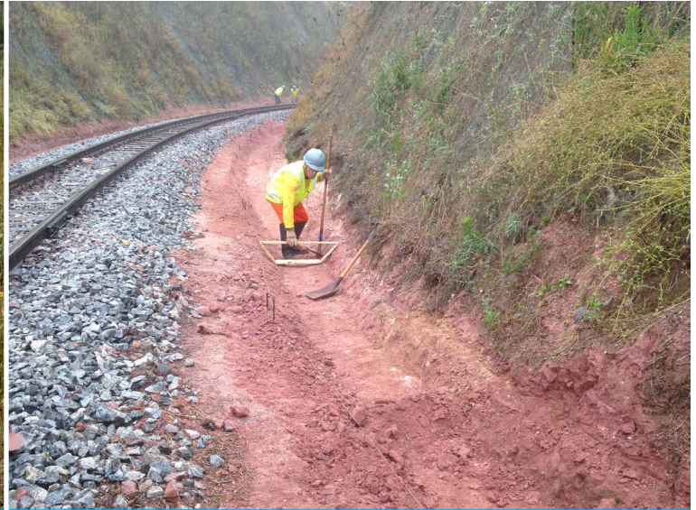
Grading the ditch
