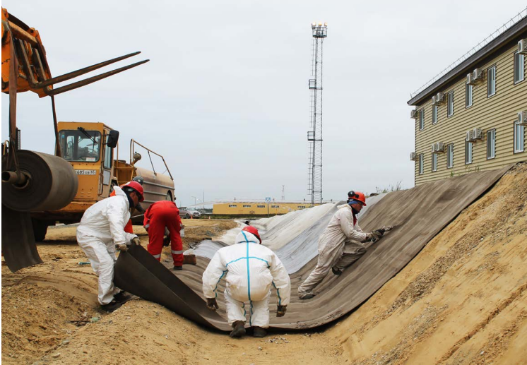
Unset CC8™ cut to length, avoiding wastage
