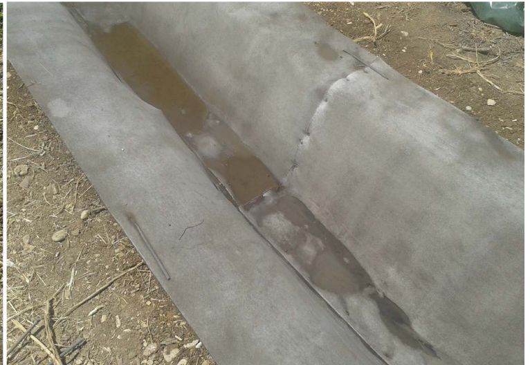
Overlapped joints
