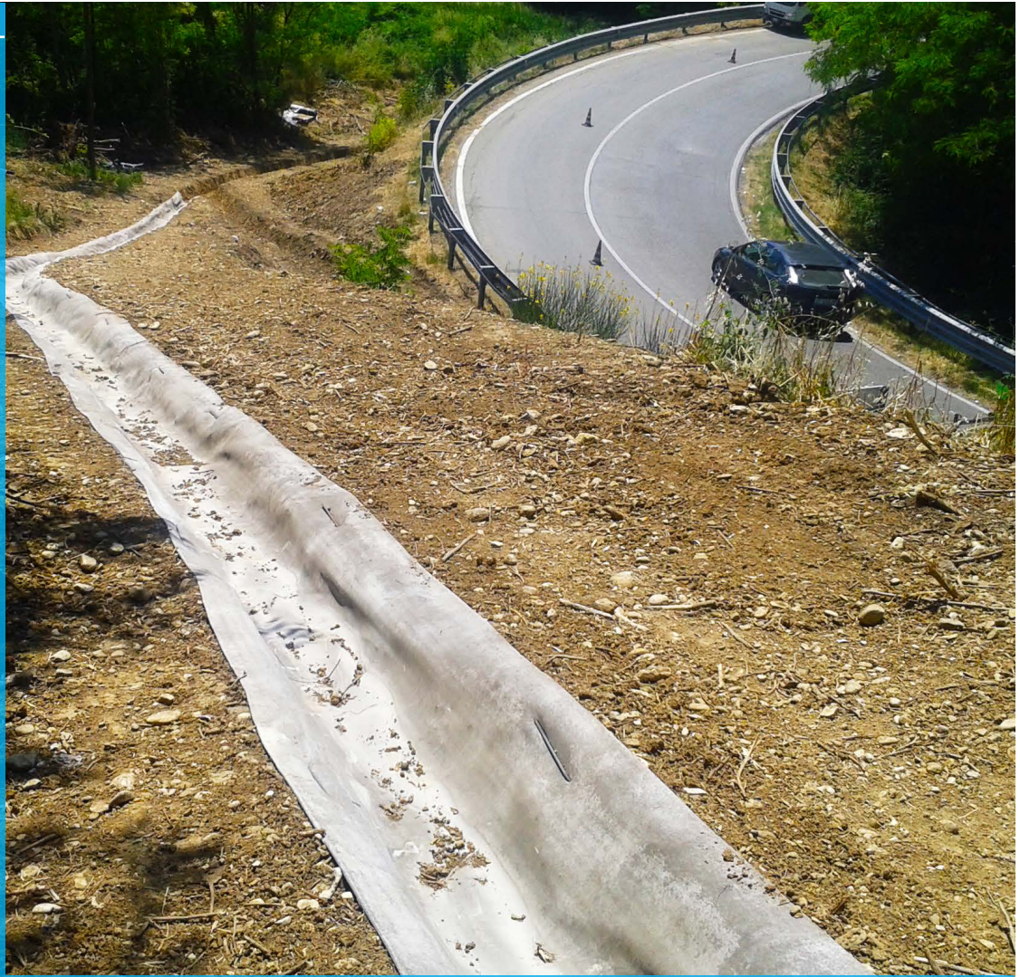
Completed section of ditch
