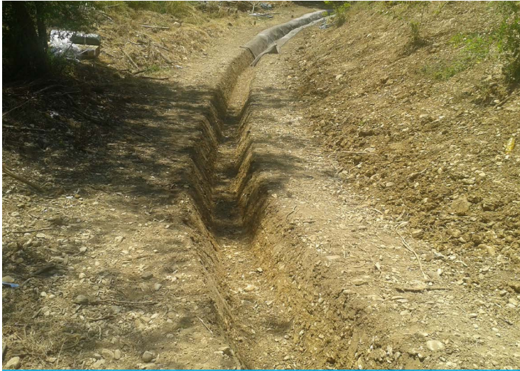
The ditch was excavated
