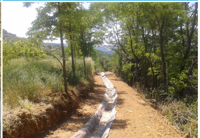
A completed section of ditch
