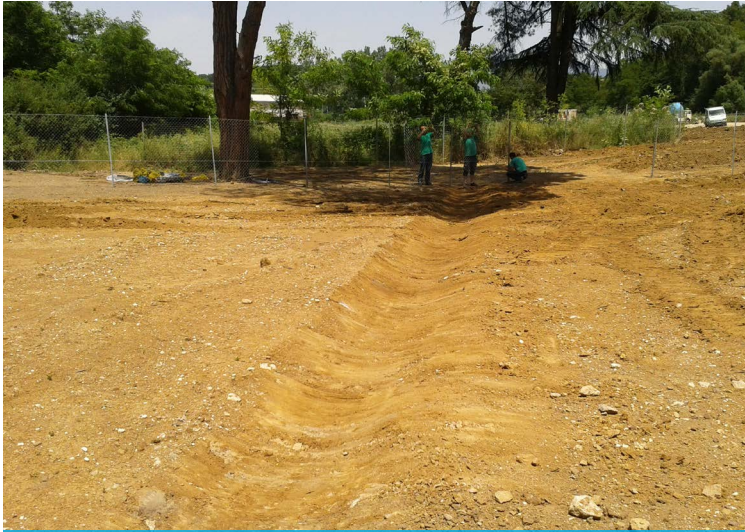
The ditch was excavated
