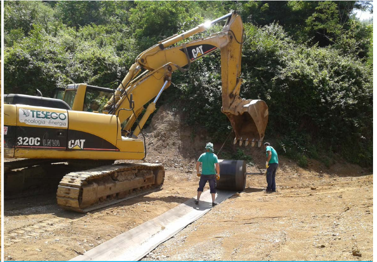
CC5™ unrolled into the ditch
