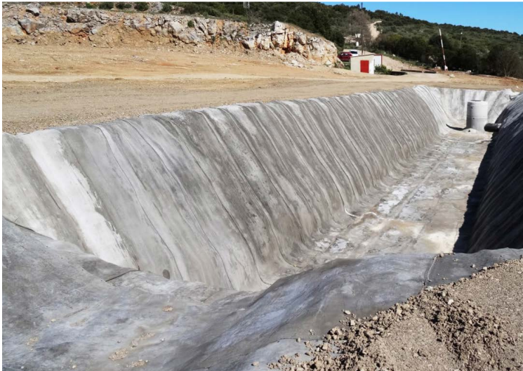
The join between the ditch and basin
