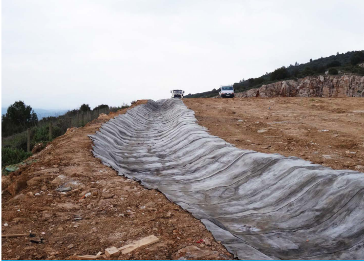
A section of the ditch
