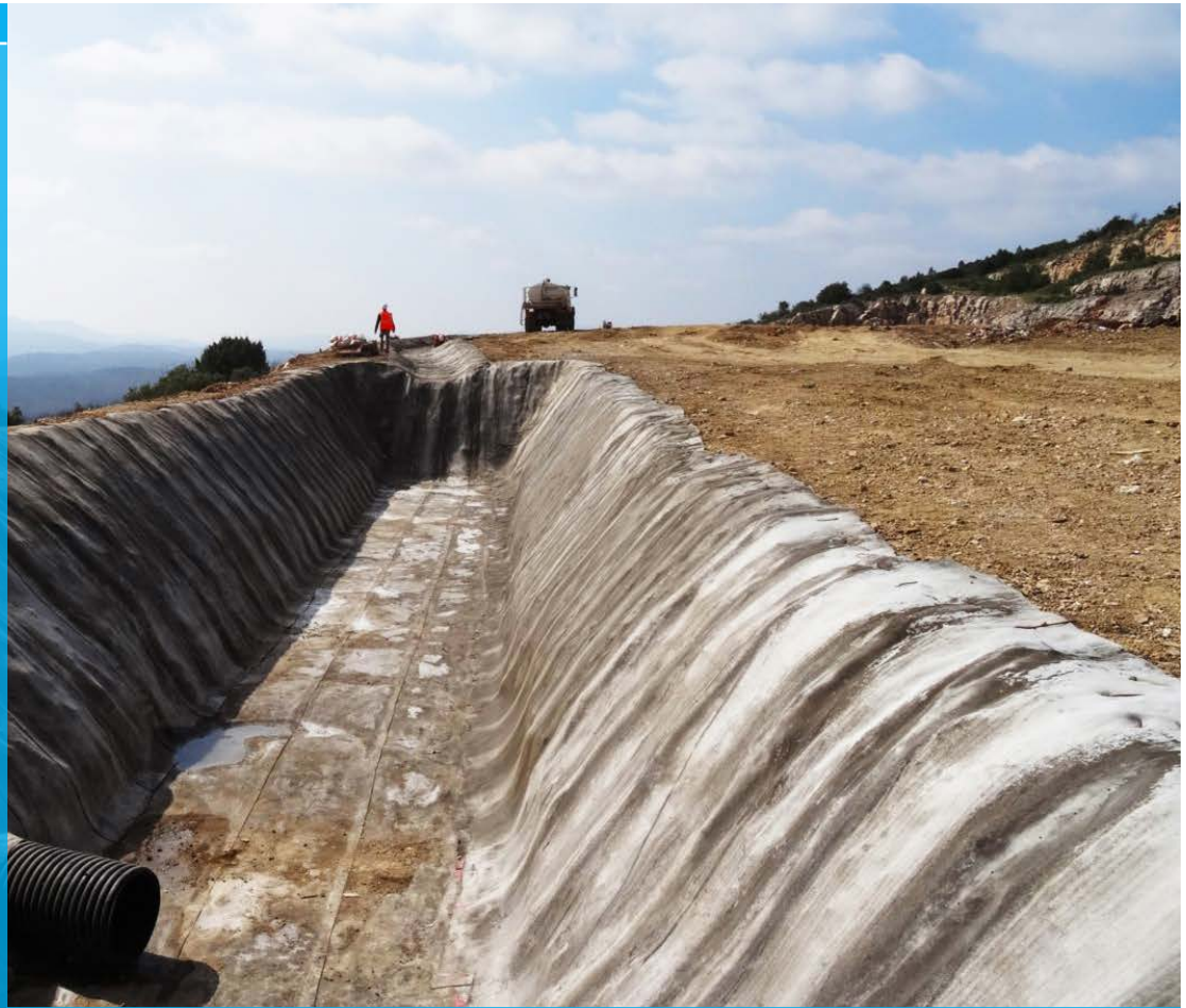
Completed basin and ditch
