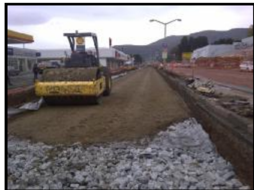
G5 sub-grade placed on reinforced layer
