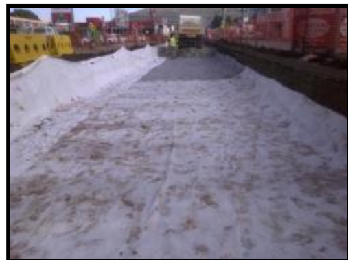
Rockgrid PC reinforcing laid in trench
