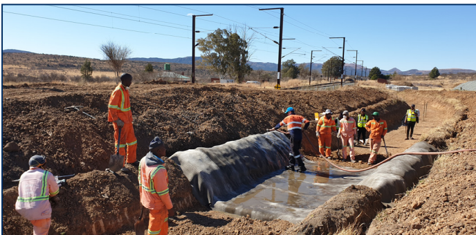
Installation - CC8 hydration process
