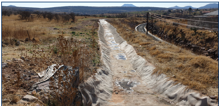
Completed northbound canal
