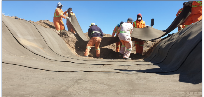
Installation of CC8
