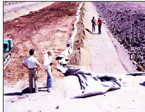
Figure 3: Mokolo Dam - Geotextile as an adjunct between core and graded filters
