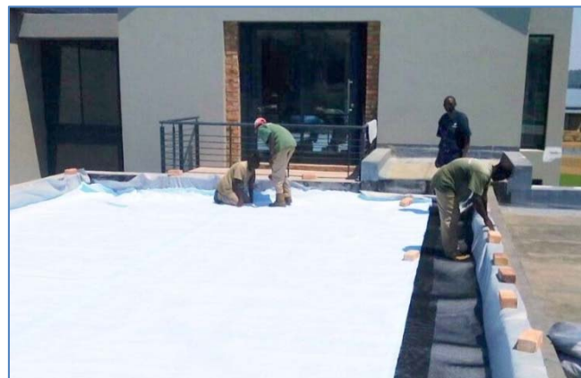
Kaytape S120 is laid over the Flownet ™
