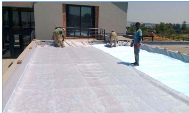
The final bidim ® A2 layer under the cover soil functions as filtration
