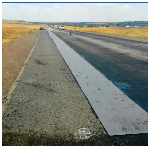
Sealmac was applied over a tack coat
