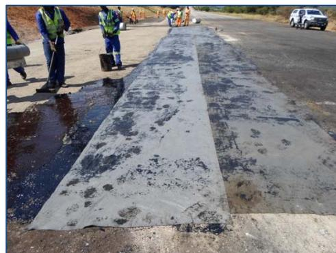
*A tack coat was applied over compacted layer works and **Sealmac**<sup>®</sup> laid on top*
