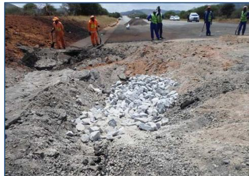
*The layer works were filled with crush run*
