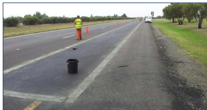
The completed temporary repair work using Sealmac ® strips
