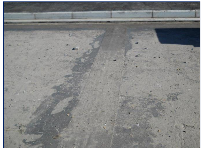
SealGrid® 50/50 placed over expansion joint.
