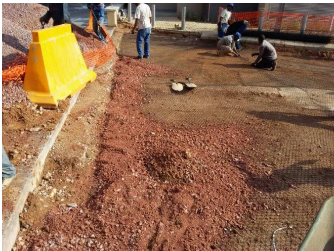
TriAx TX160 was laid and overlapped by 300mm before end-tipping G5 on it
