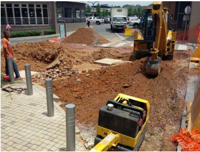
The paving was removed and existing fill excavated to 300mm depth.
