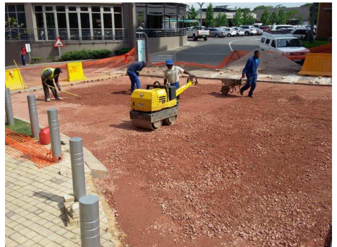
The G5 material was spread and compacted before relaying the paving.
