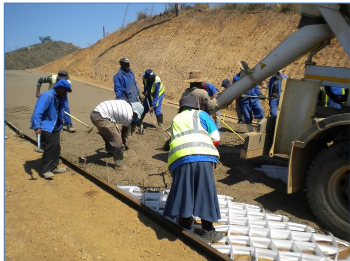
Local community labour with basic training, was used to install Multi-Cell®
