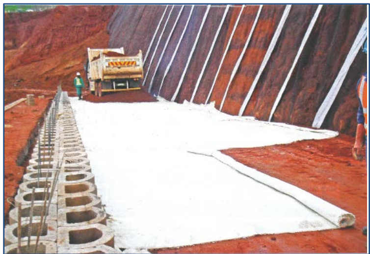
The Terraforce walls once completed, with the reinforcement of RockGrid® PC
