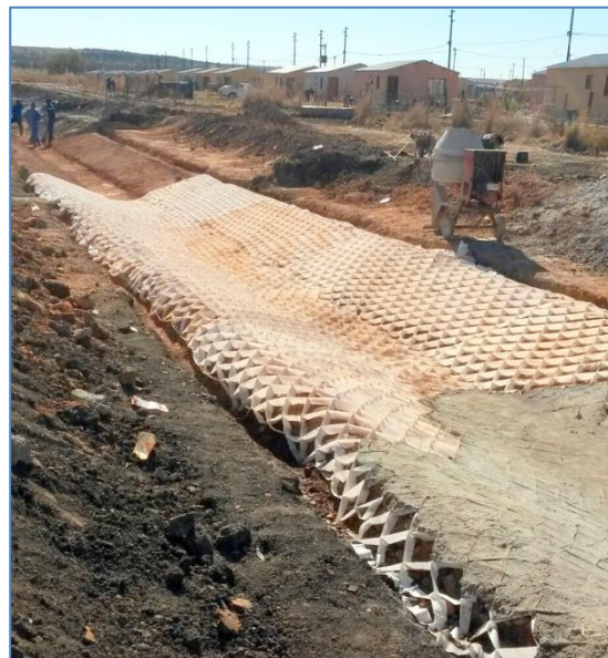
Multi-Cell ® was laid along the canal and into the anchor trenches
