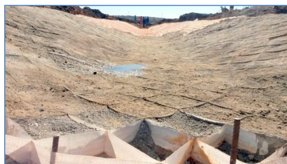
Reinforcing Multi-Cell ® was filled with concrete
