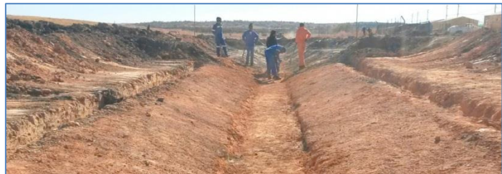
anchor trenches dug at crests of the canal
