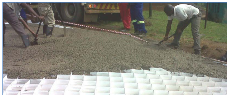
Multi-Cell® was filled with concrete
