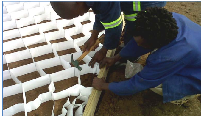
Multi-Cell® was easily installed using local labour
