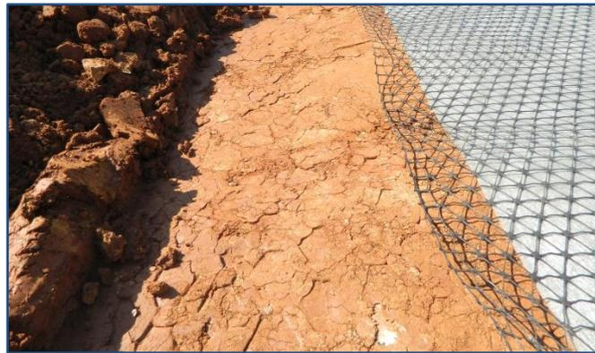
*The low bearing capacity substrate was compacted.*
