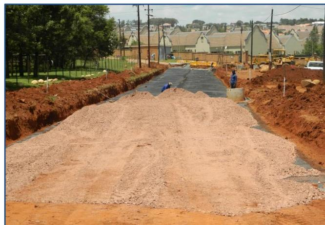
*First cover layer is placed directly over TriAx<sup>™</sup>.*
