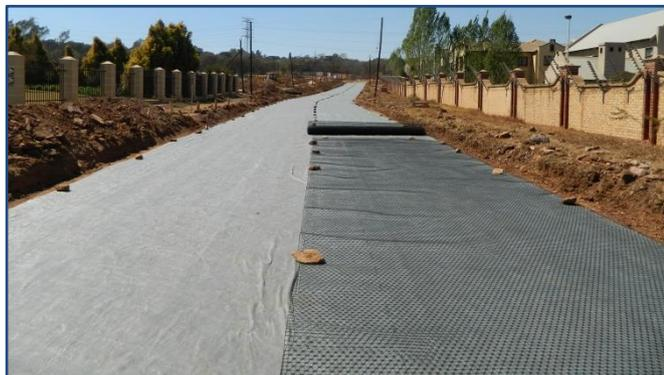
*TriAx<sup>™</sup> placed over the separation layer.*
