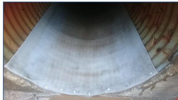
Concrete Canvas was pop-riveted to the existing steel culvert
