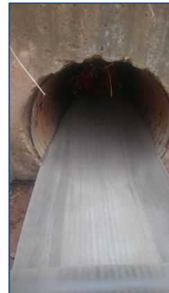
Concrete Canvas was manually pulled through the culvert
