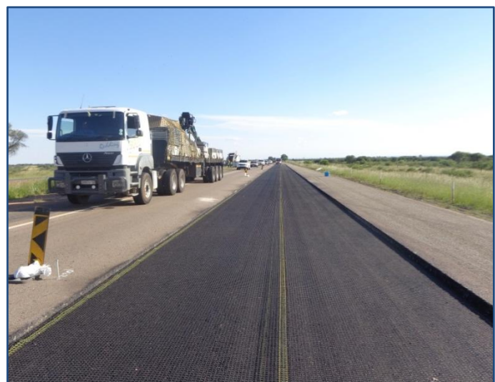
Glasgrid ® laid over roads to effectively reinforce the asphalt layer.
