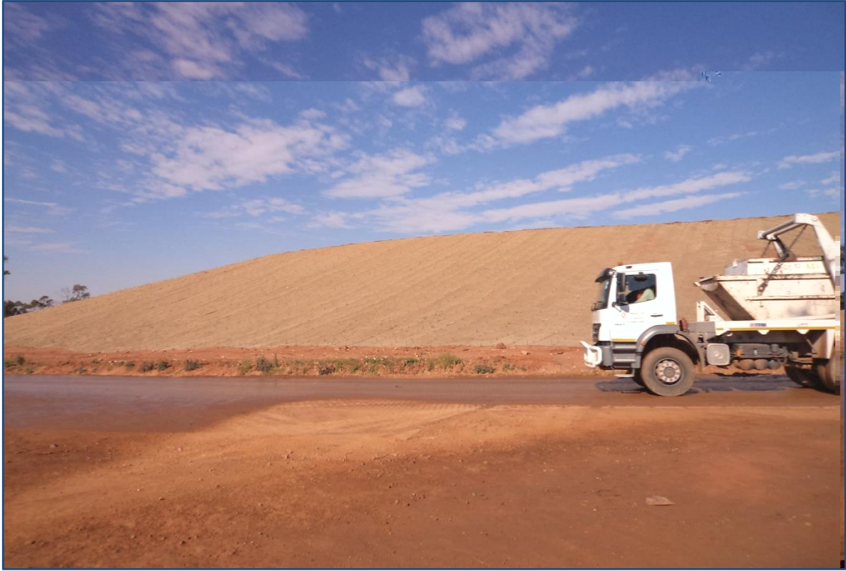
Luipaardsvlei Landfill slope covered by SoilSaver ® , ready for grass re-growth.
