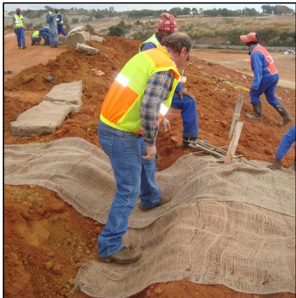
Laying SoilSaver® in the anchor trench
