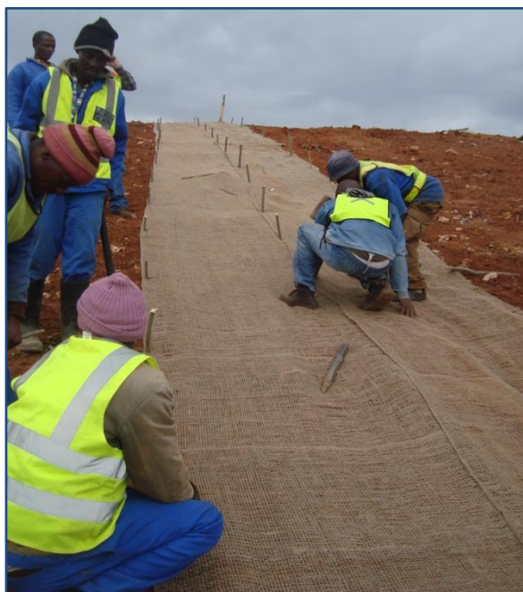
SoilSaver® edges are overlapped and held in place with wooden stakes.
