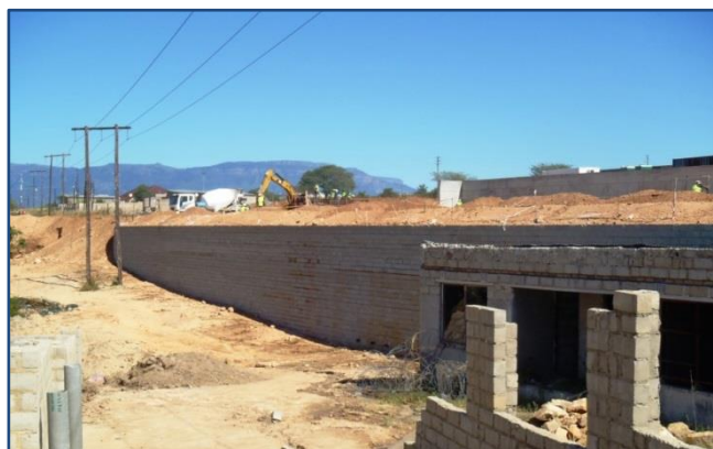
The reinforced retaining wall at Acornhoek Shopping Centre.
