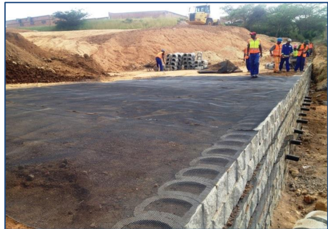
Miragrid GX 75/75 and used to reinforce the retaining wall.
