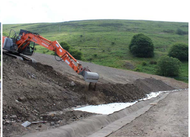
Burying the CC and geosynthetic
