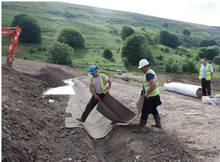
Positioning the CC in the ditch
