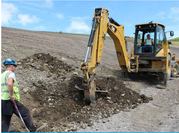
The ditch was excavated to profile
