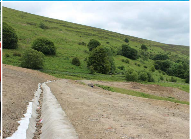
A finished section of ditch
