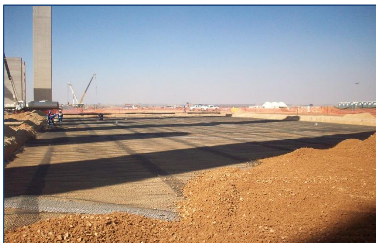
35 000sqm of TriAx™ evens out the load on the loading platform.
