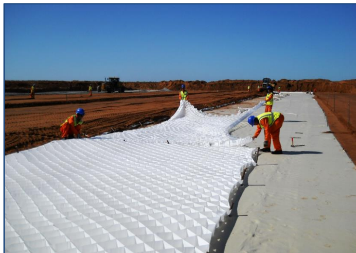
Multi-Cell® and RockGrid® PC were used to reinforce the access road.
