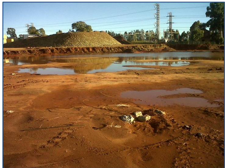
Heavy rains and a mix of in situ material rendered conventional reinforcing methods ineffective.
