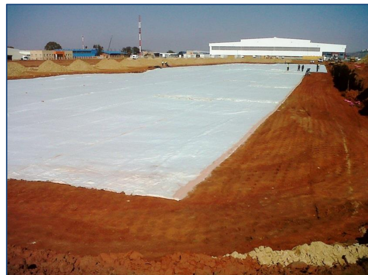
29000sqm of Rockgrid® PC was used to reinforce the substrate.
