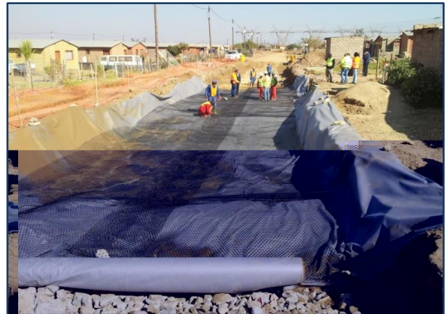
TriAx™ TX160 laid over geotextile separation layer
