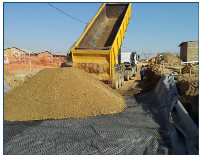
350mm of G5 material placed over TriAx™
