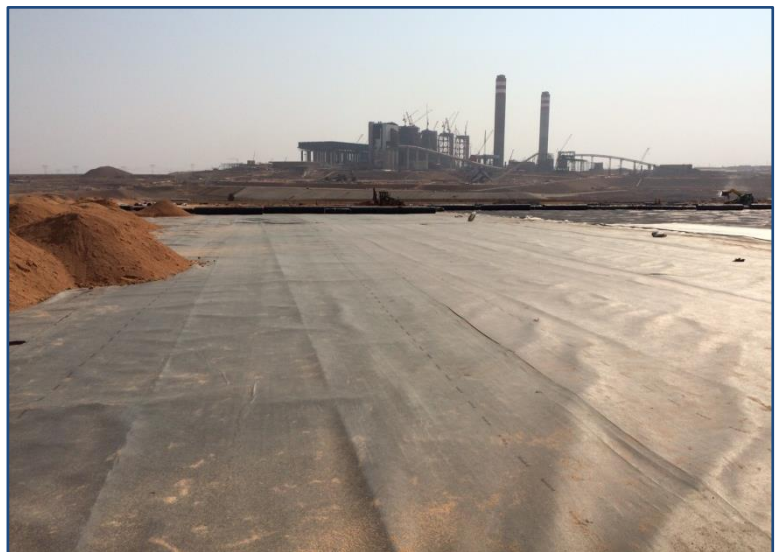
750gsm geotextile laid out to be covered with sand
