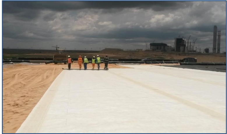
EnviroFix® X1000 GCL laid over sand
