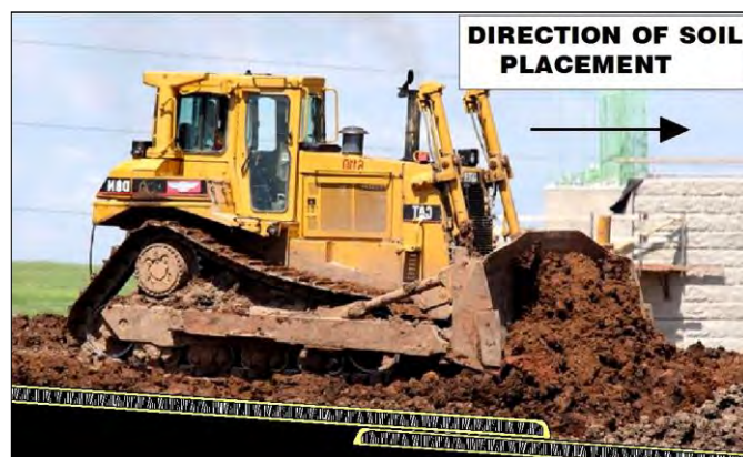
Figure 20: Covering soil placement
