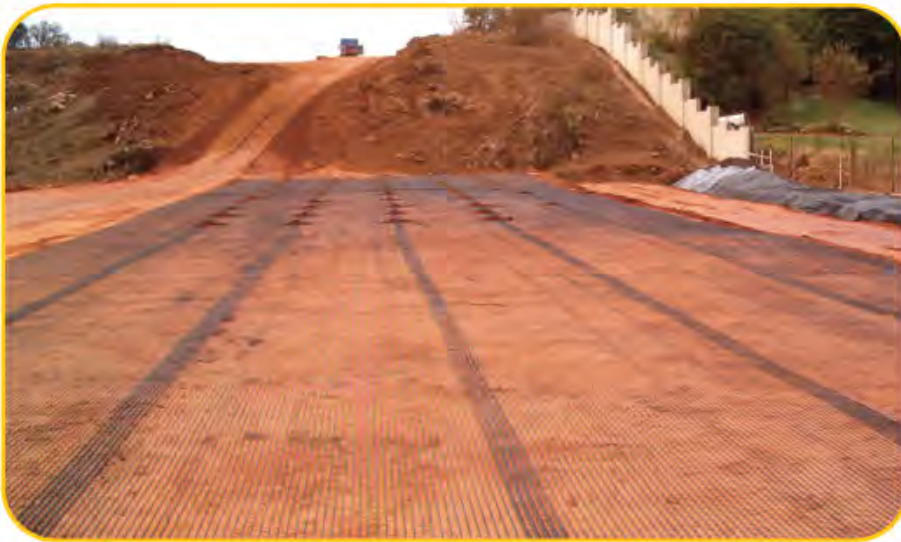
Left: Insufficient interlocking of stiff extruded geogrids
