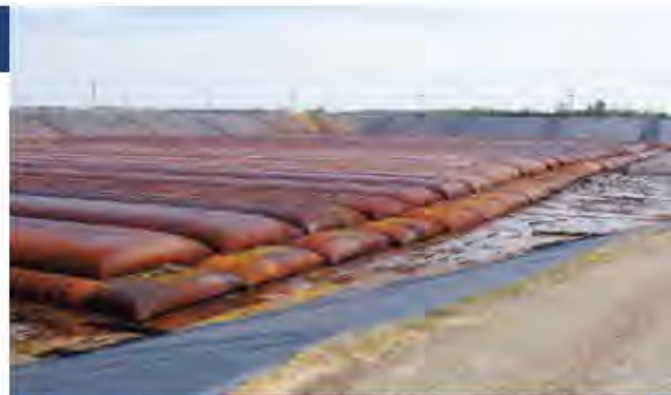
Coal sludge dewatering using Geotube® dewatering technology
