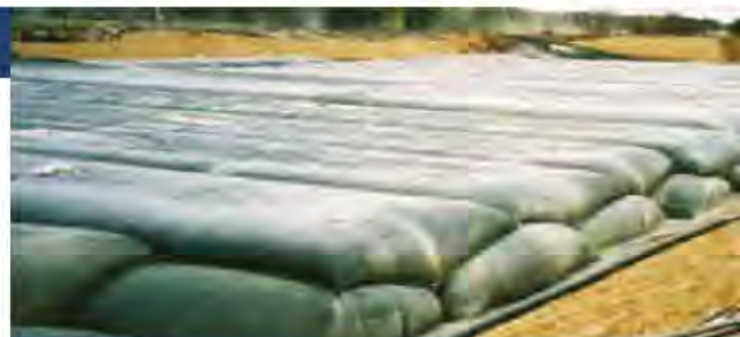
Geotube® containers in activated sludge basin at paper plant
