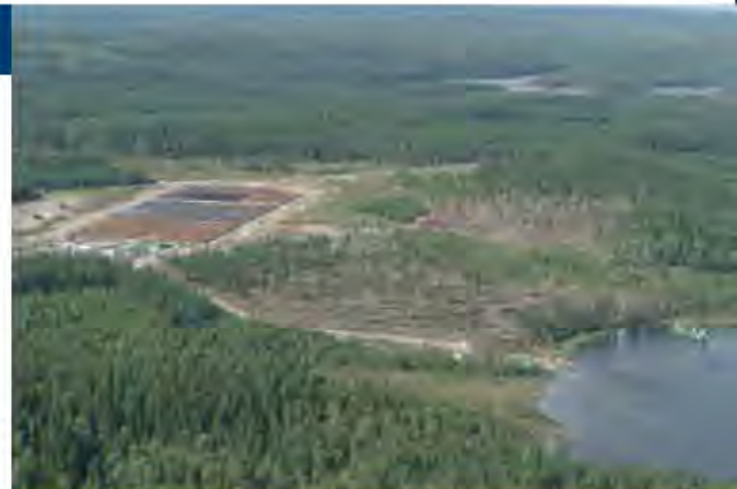
Geotube® containers prevent contaminated run-off from entering the local lake.
