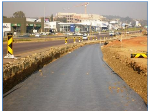
bidim ® A2 laid as separation
