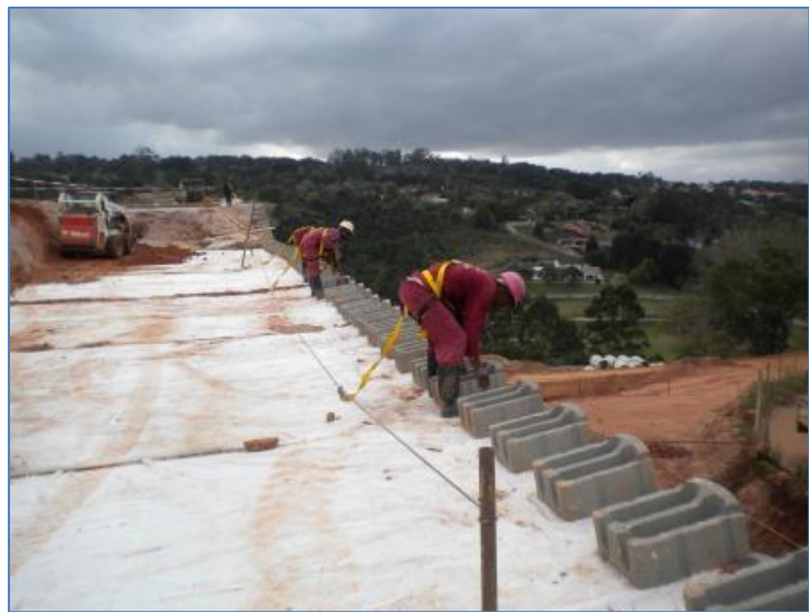
Rockgrid® PC was laid at every third row of blocks
