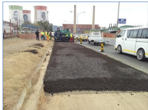
200 mm ETB and 40 mm asphalt cover the TriAx ® mechanically stabilised layer
