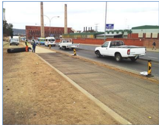
Laying down TriAx ® TX170
