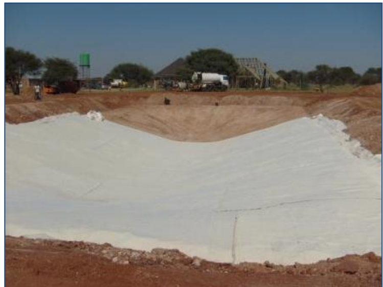
EnviroFix® was laid to prevent leaks
