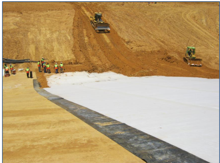
EnviroFix® GCL was easily laid on the steep slope
