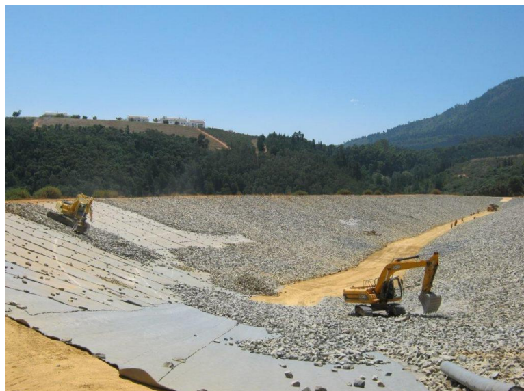
bidim® A8 forms a protection layer with the riprap
