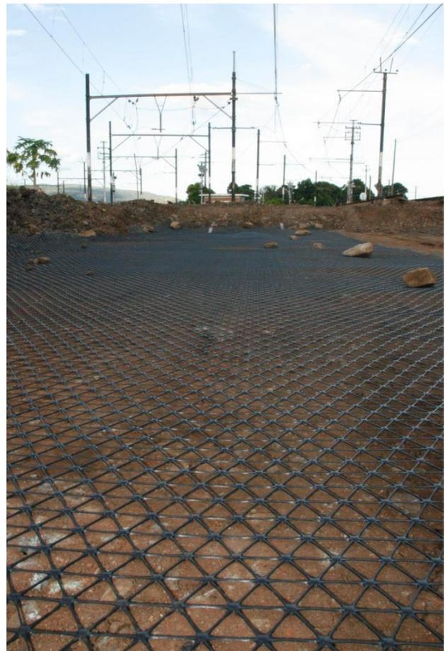
Picture 1: TriAx™ TX160 being installed
