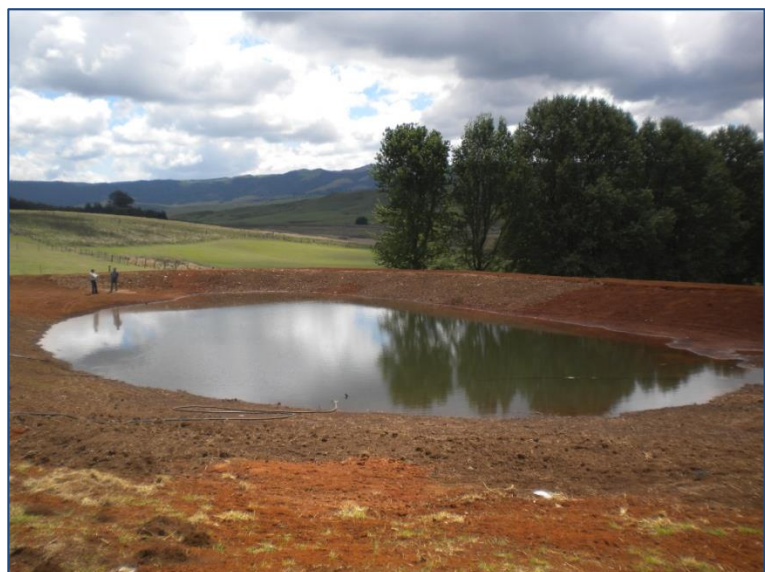
Filling the completed dam lined with EnviroFix® GCL
