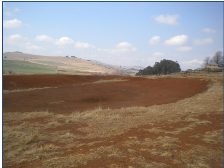
The new dam slopes prepped for lining
